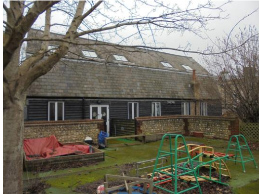
Southern elevation of the Tithe Barn and walled garden
