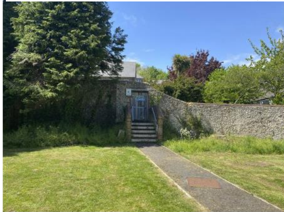
Fig. 4.7: A recent flint and brick staircase with modern treads.
