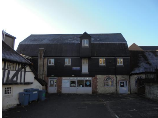
Northern elevation of Tithe Barn
