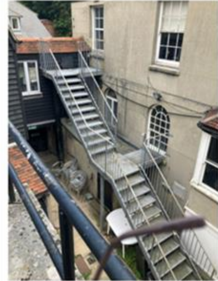
Fig. 4.46: Part of the Victorian extension to the Manor House as seen from the internal courtyard, with the fire escape.
