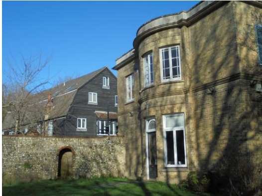
1913 wing of the Manor House and adjacent flint wall
